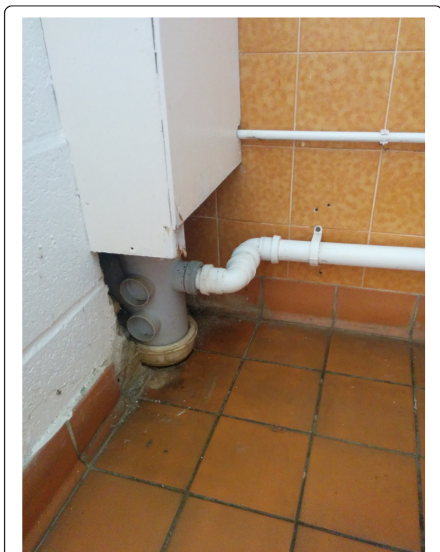
Fig. 1 Photograph showing the primary collection area of resting mosquitoes in the toilet block at Elmley. Blood-fed Anopheles maculipennis s.l. mosquitoes were found resting directly on the walls and on or under the exposed wooden covering to the pipework
